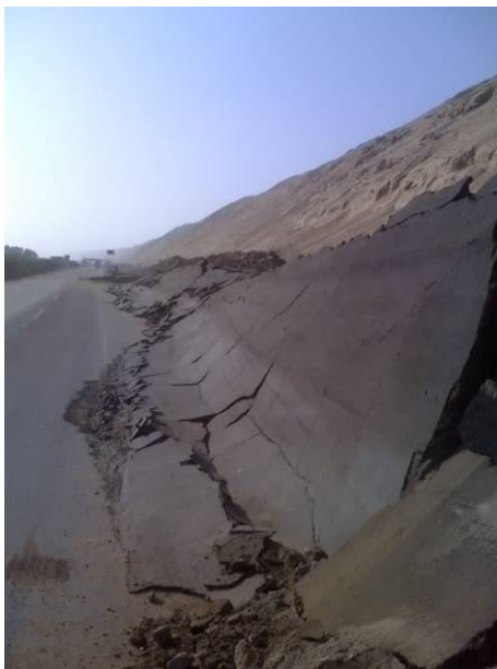
Fig. 5.8 Lifted shoulder at Playa Jahuary. South Pan-American Highway
