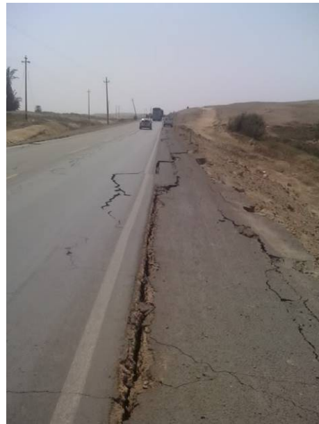
Fig. 5.5. Shoulder settlement and displacement
