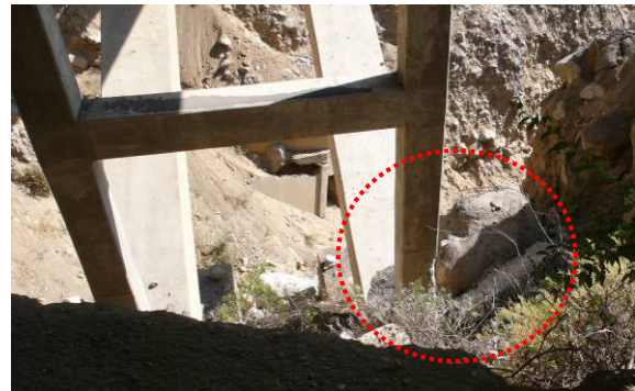
Fig. 5.15 Rock impacted on bridge substructure (Tsej Tji Bridge, Los Libertadores Highway, close to Huaytara)
