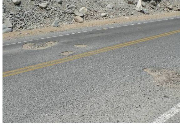
Fig. 5.6. Road distortion due to liquefaction Fig. 5.7 Pot holes caused by rock falls induced lateral spreading
