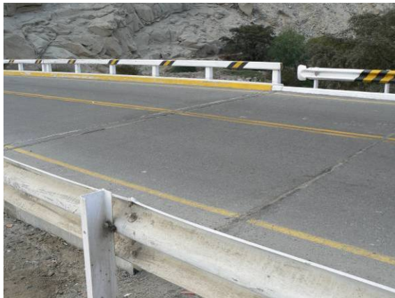
Fig. 5.14 Mild settlement of the fill behind abutment (La Quinga Bridge, Los Libertadores Highway)
