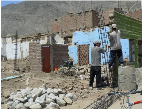
Fig. 6.11 Front adobe wall, which did not collapse during the earthquake, is reused in the new structure with some “reinforcement”
