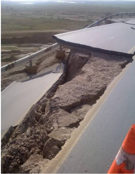
Fig. 5.2. Slope failure caused by liquefaction induced lateral spreading
