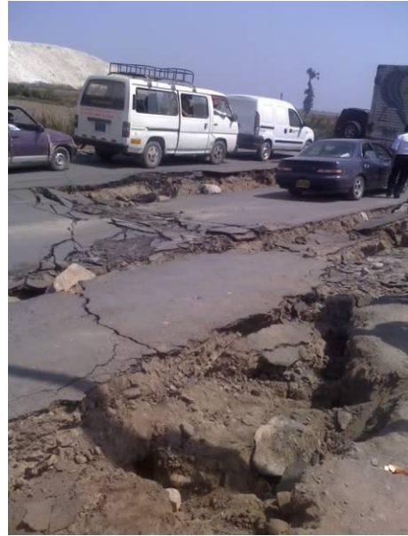
Fig. 5.3. Liquefaction induced embankment failure
