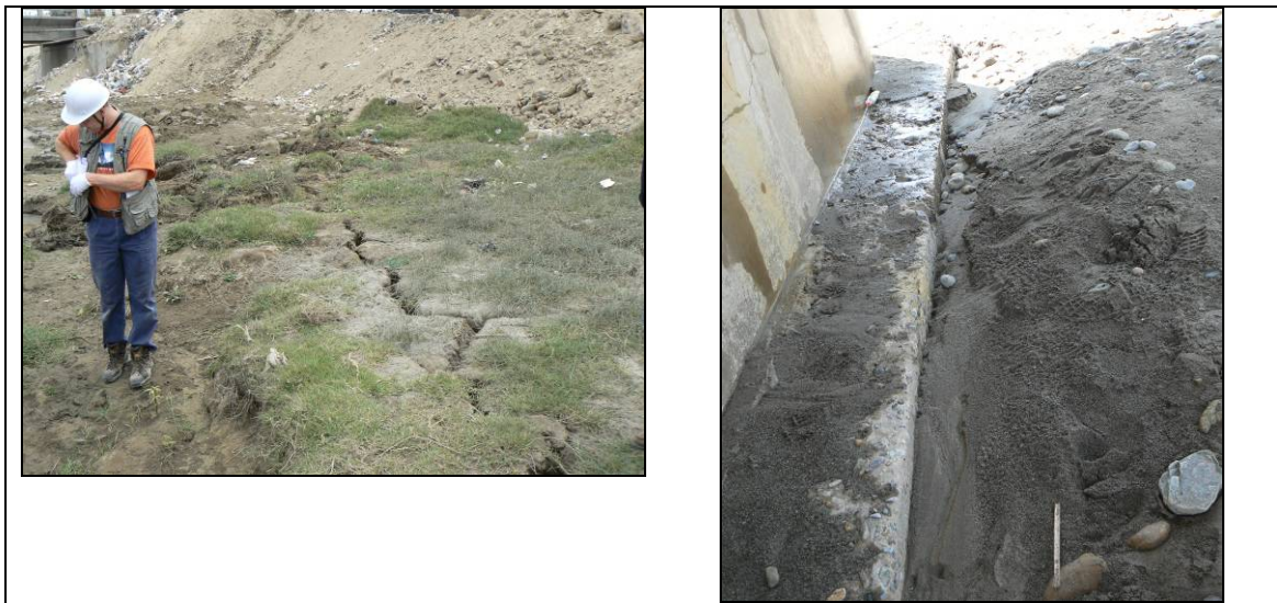
Fig. 5.18 Liquefaction induced lateral spreading (Pisco River north upstream pillar bank)
