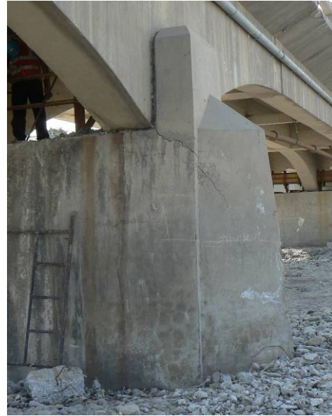
Fig. 5.30 Cracks in the wing of the pillar with fixed bearing
