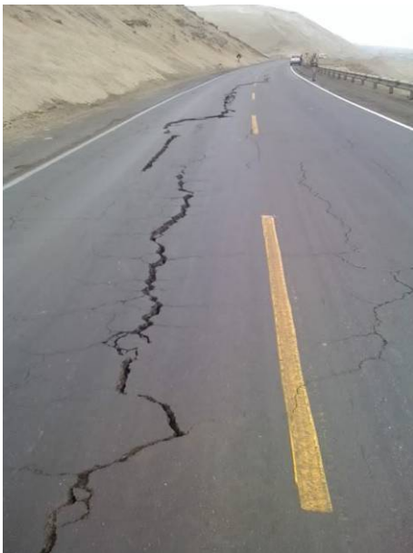
Fig. 5.4. Cracking along the pavement due to landslide induced movement
