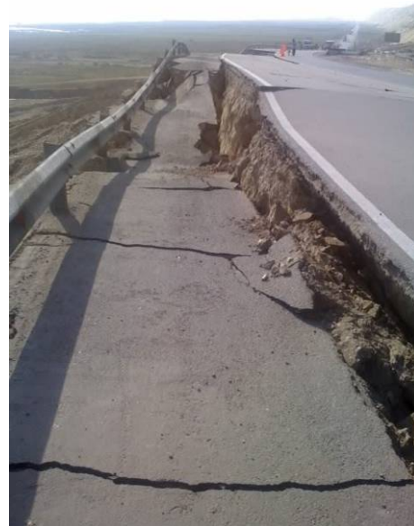
Fig. 5.9 Road failure due to lateral spreading at the foot of the slope. South Pan-American Highway
