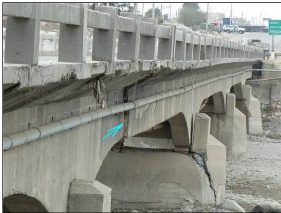
Fig. 5.25 Bridge slab displacement (picture taken towards the north). Arrow indicates the gap corresponding to the southern 8 cm gap shown in Fig. 5.24
