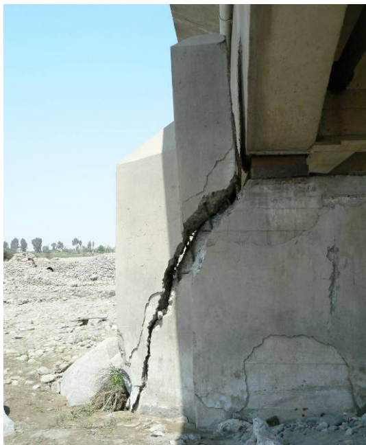
Fig. 5.27 Failed wing with poor reinforcement (pillar with movable bearing)
