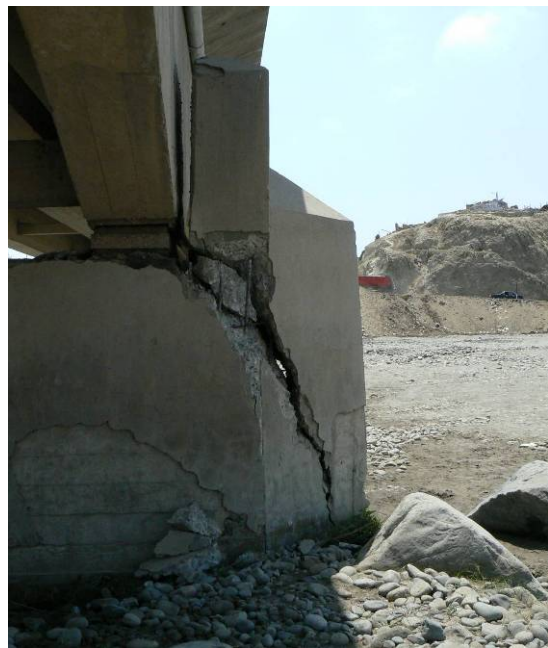
Fig. 5.28 Failed wing with poor reinforcement (pillar with movable bearing)
