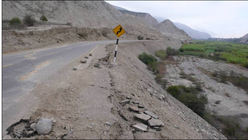
Fig. 5.12. Slope failure at Canete-Yauyos road (Km. 23)
