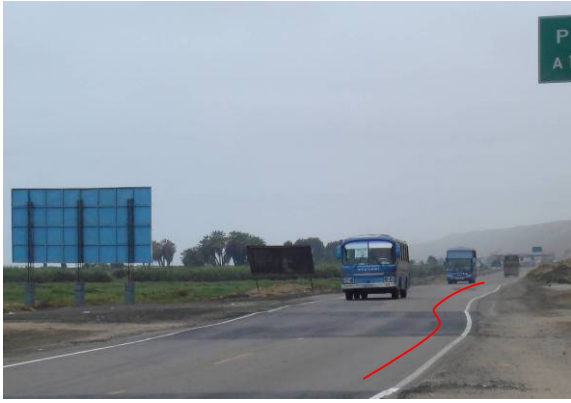
Fig. 5.6. Road distortion due to liquefaction Fig. 5.7 Pot holes caused by rock falls induced lateral spreading
