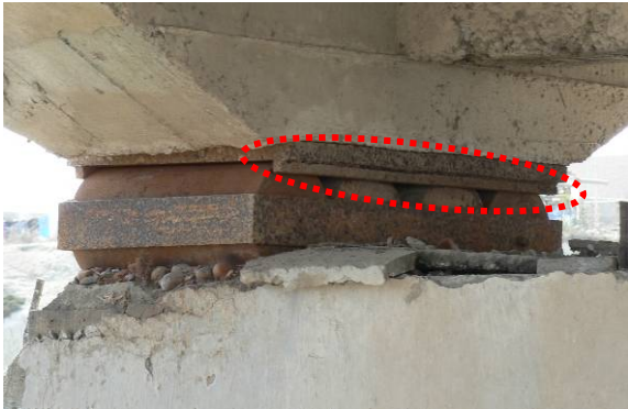
Fig. 5.22 Movable bearings on the pillars
