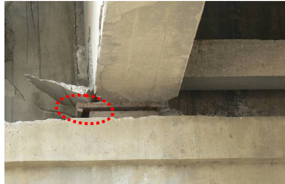
Fig. 5.23 Movable bearing at the southern abutment
