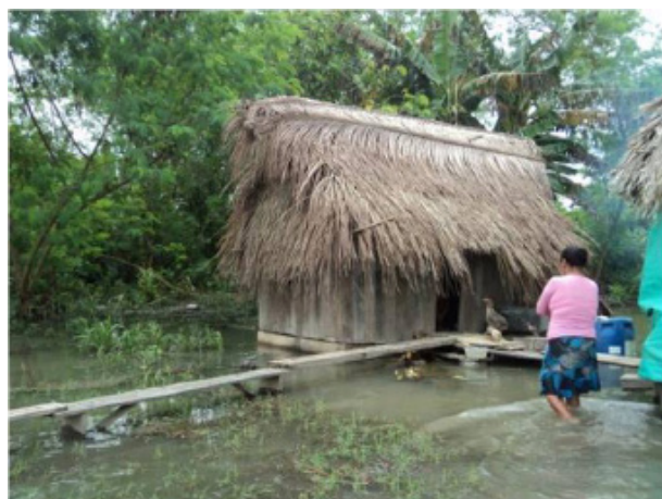
Poultry house affected by flood
