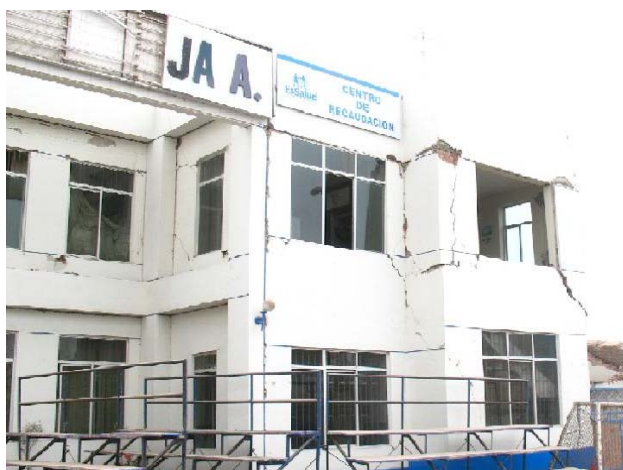
Hospital de ESSALUD
